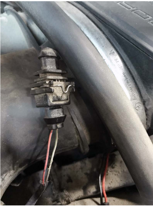
Pictured Left: Find a key hot 12V power source to tap into. Cut back any heat shielding/wrap to expose the wires.
